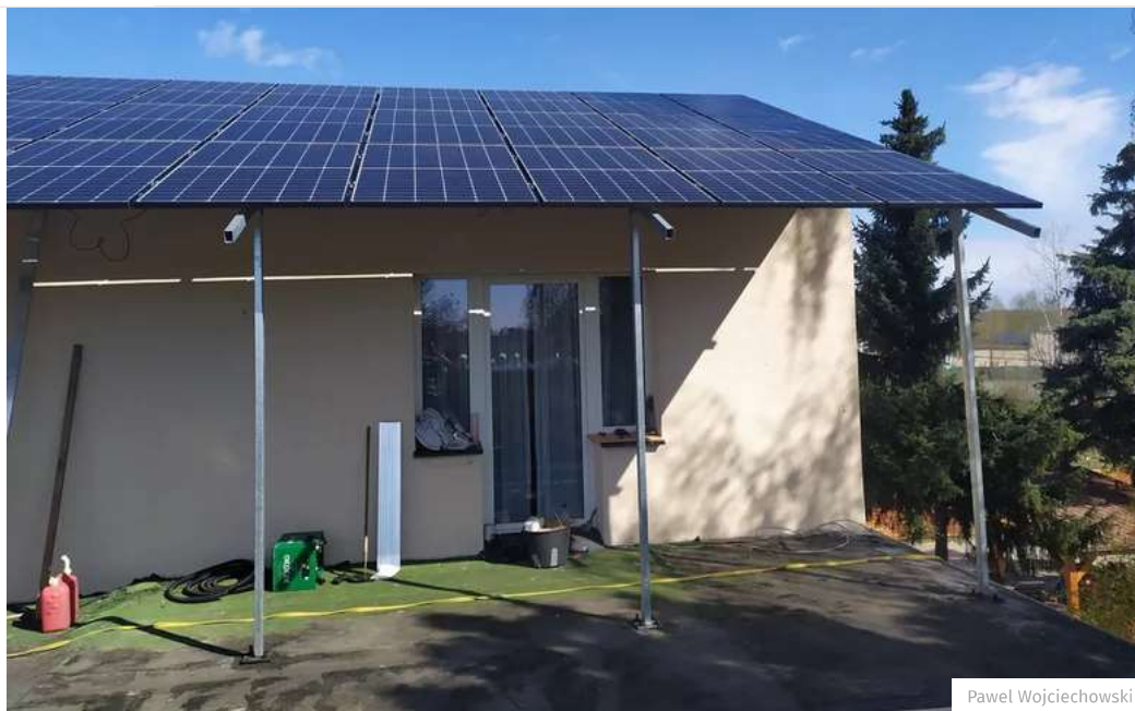
The first part of Paweł Wojciechowski's photovoltaic installation
